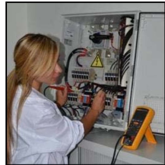
Insulation test @ 1,000V
